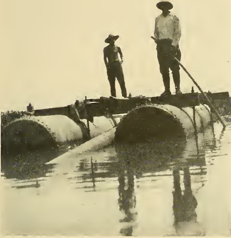
FLOATING THE PIPE LINE ACROSS THE RIVER
